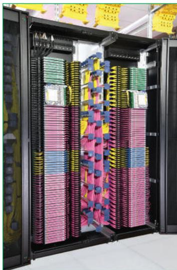
*Fig. 1: Fibre management systems are crucial in organising the cabling in a clear and concise way, reducing the risk of damage and downtime.*
