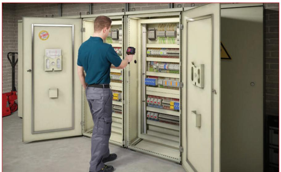
Fig. 1: A thermal imager can detect anomalies such as overheated connections in a control cabinet.
